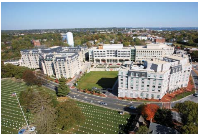
Park Place - Project included construction of 3 level below grade parking garage, Westin Hotel, 250 plus high end condos, 2 separate office buildings. liti-use
